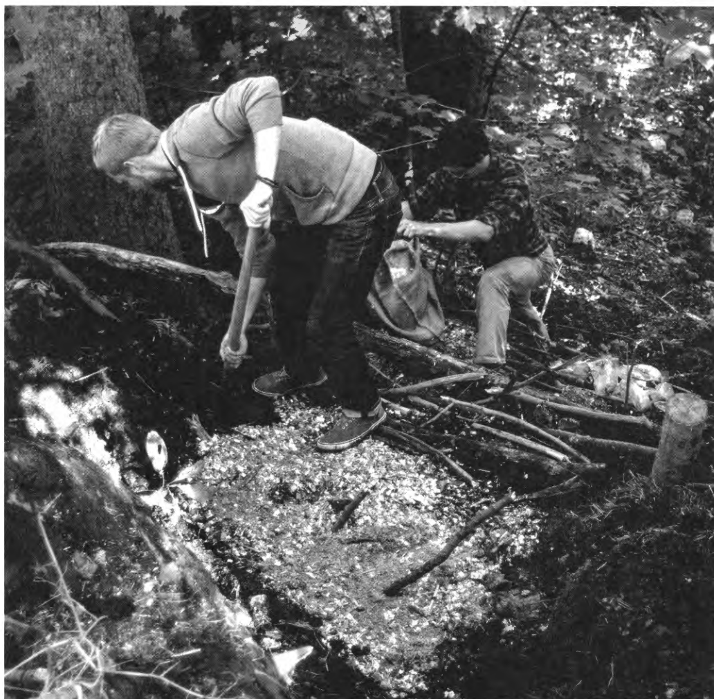
A two-tiered microbial filtration system, designed by the author, being installed in western Massachusetts. The target pollutant was effluent overflowing from an antiquated septic system.
