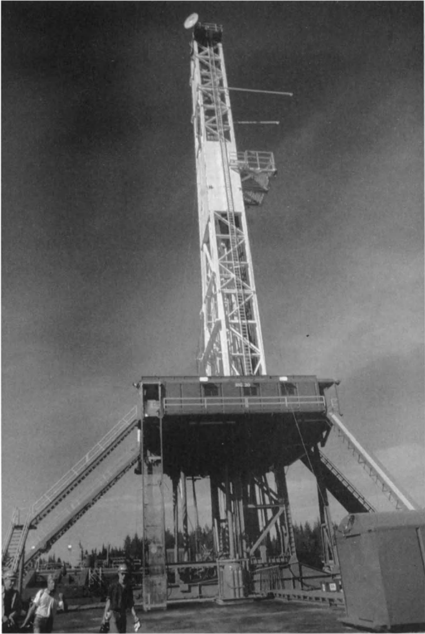
Figure 6.4 Site of the drilling project in the Siljan Ring.
